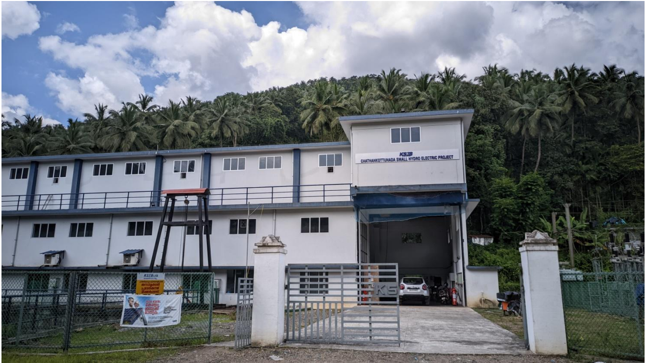
Chathankottunada II SHEP commissioned on 21.06.2021
